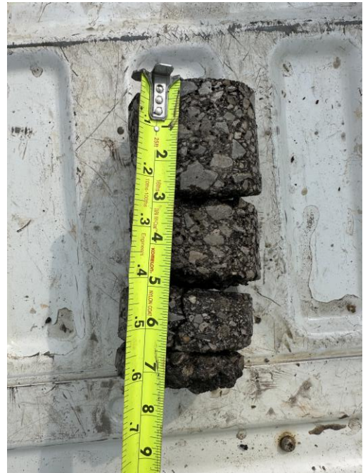
Asphalt Core C-06
