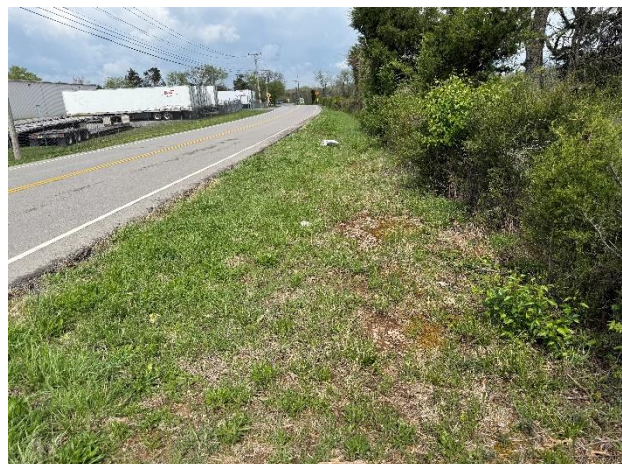
View of Epps Mill Road looking north towards its intersection with SR2
