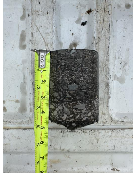
Asphalt Core C-02
