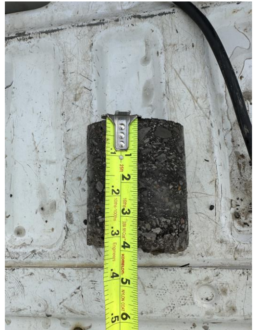
Asphalt Core C-04
