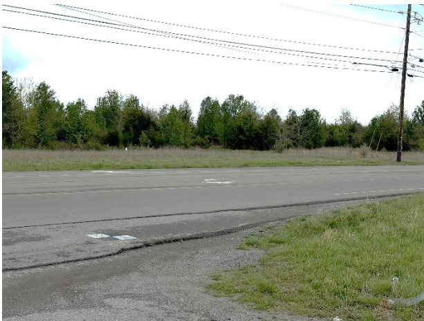
View of Epps Mill Road near its intersection with Capital Way
