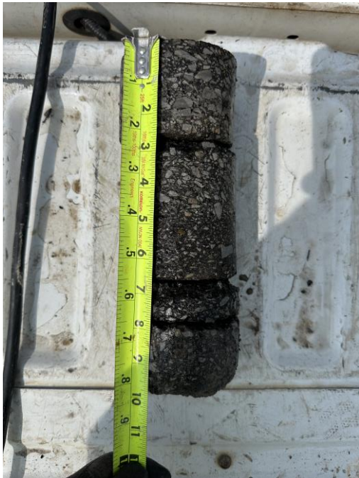
Asphalt Core C-05
