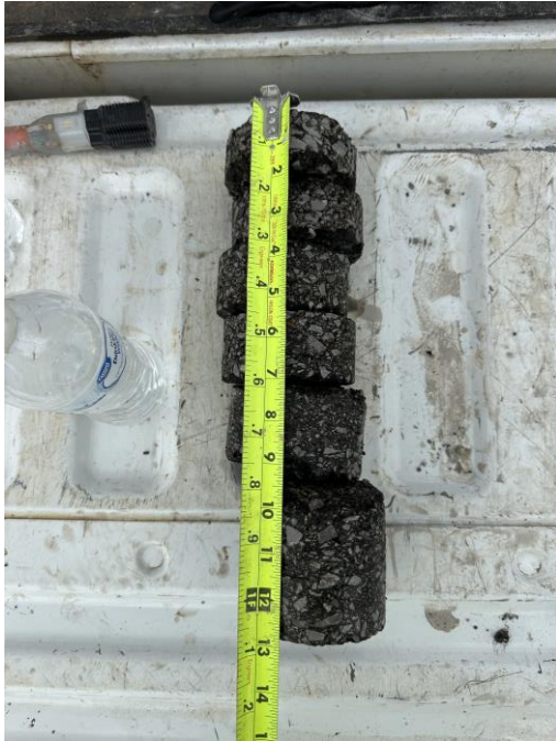
Asphalt Core C-01
