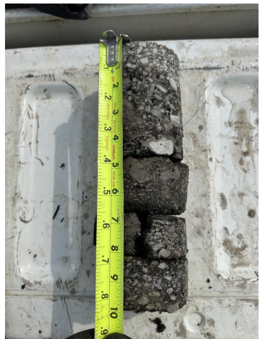
Asphalt Core C-08
