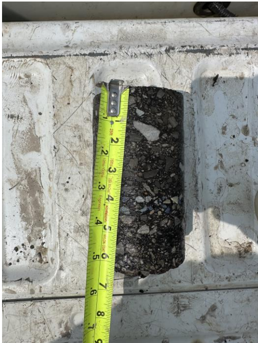
Asphalt Core C-03
